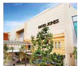
David Jones Building Retail
