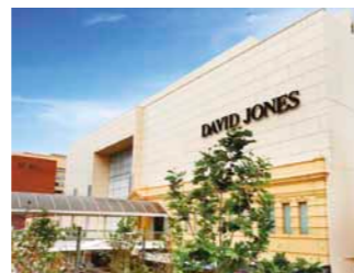
David Jones Building, Murray Street
